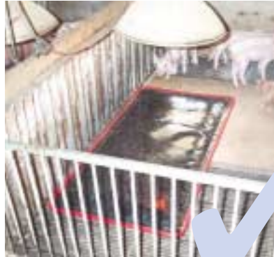
Meeting Rule 1: Example of an open pen wall made solid.
